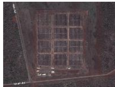
1.2 MW PV Plant
