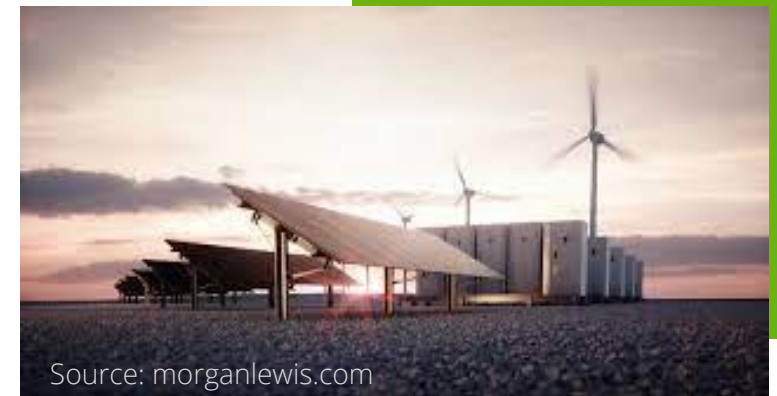
RENEWABLES PLUS STORAGE
